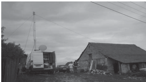
Figure 5 Instalment of mobile base station TETRA in Obrenovac (Source: MoI Republic of Serbia)
