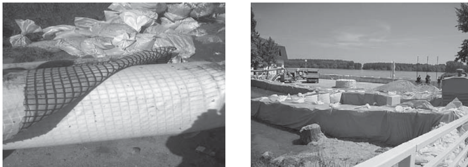
Figure 3 Impermeable foil for ensuring primary embankment and box barriers used for constructing embankments
